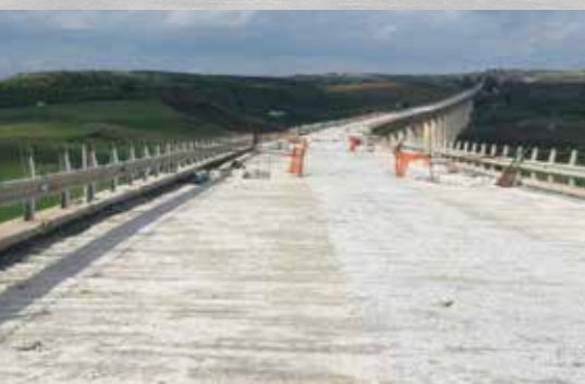
ssi bridge / italy
