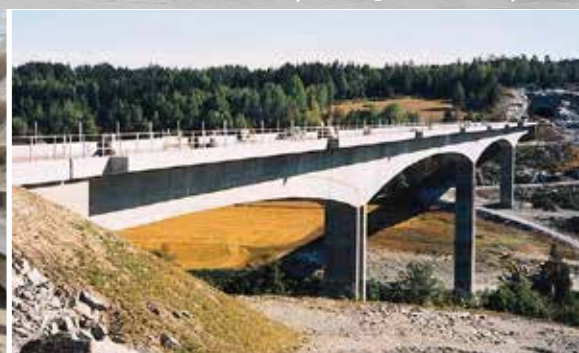
Holendalen railway bridge / Norway
